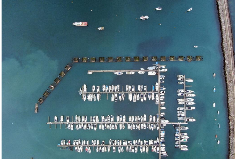
Figure 10. The 22 platform that make up the wave barrier at MDL Marina Brixham, South Devon. Duncan Kenny. 2024.
